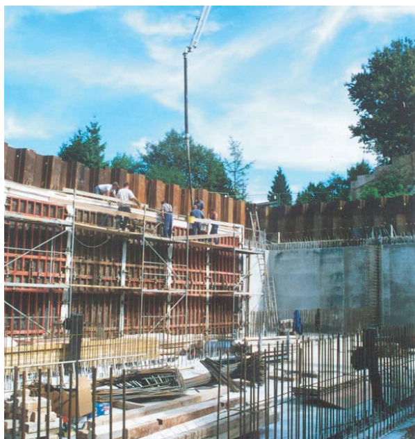
Casting of the west-wall
