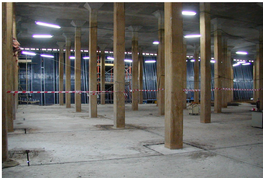
Figure 1: The construction site of Water Service Reservoir
