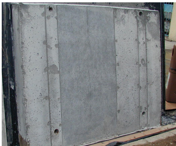
Figure 2. A trial for installation of Formtex ® (middle)
