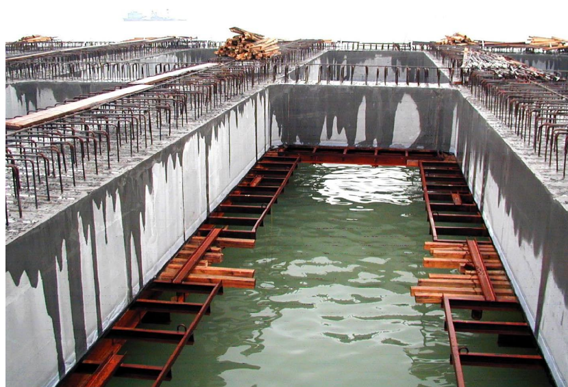
Figure 1. The construction site at Shekou Container Terminals.
