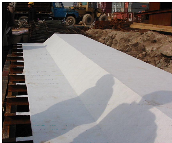
Figure 3. Formtex is easily glued onto the angular Steel formwork.
