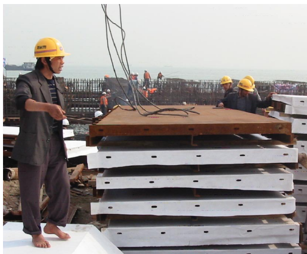
Figure 2. Formtex ® is efficiently installed on the steel formwork.
