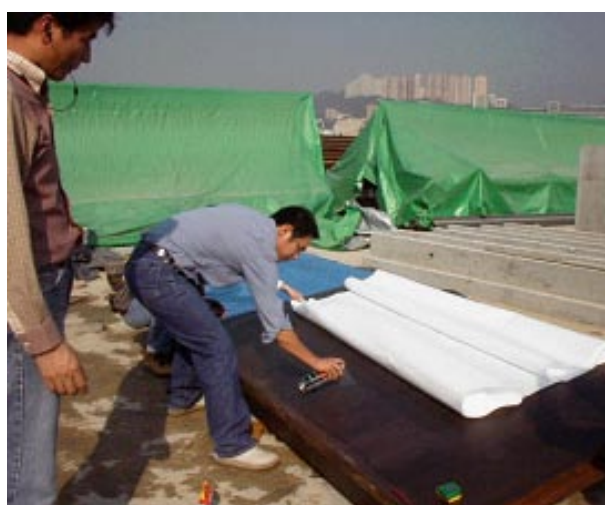
Figure 9. Test formwork is prepared with the competing product on the left and Formtex ® on the right.
