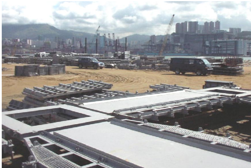
Figure 1. The construction site at Container terminal No. 9.
