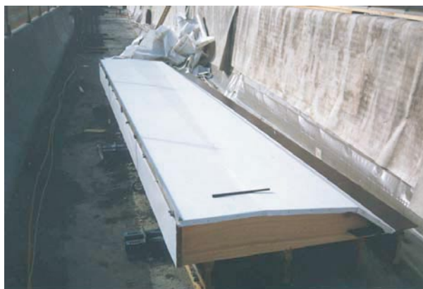
A formwork element lined with Formtex ® ready for casting.
