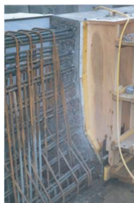
Casting of parapet and finished result.
