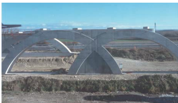
Bridge parapet cast with Formtex ® .
