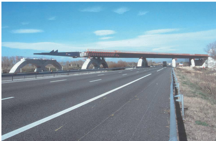
Railway bridge for French TGV high-speed trains crossing the RN9.
